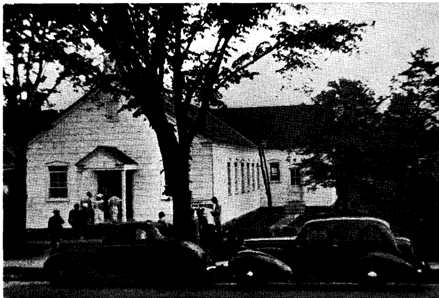
New home of Calvary Church, Wildwood. The wing in the rear is part of the Sunday school quarters. In Wildwood water begins not only at the beach, but a few feet down anywhere: with a basement out of the question, the Sunday school auditorium is at the back of the T-shaped edifice.
