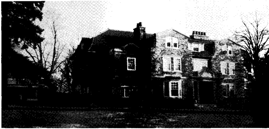
OPC Administration Building
